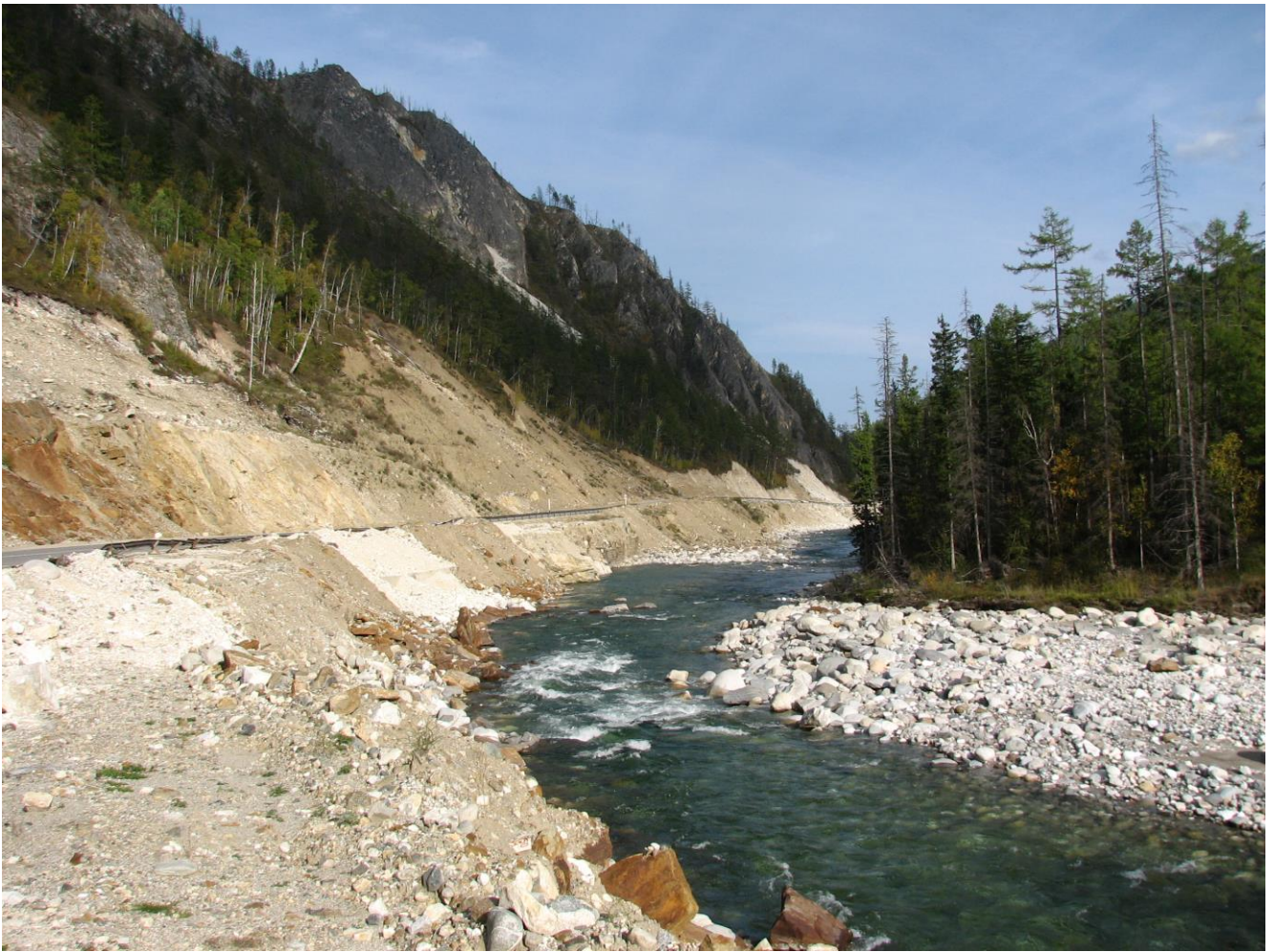
The road from Kyren town to the Mondy village along the Irkut River valley.
